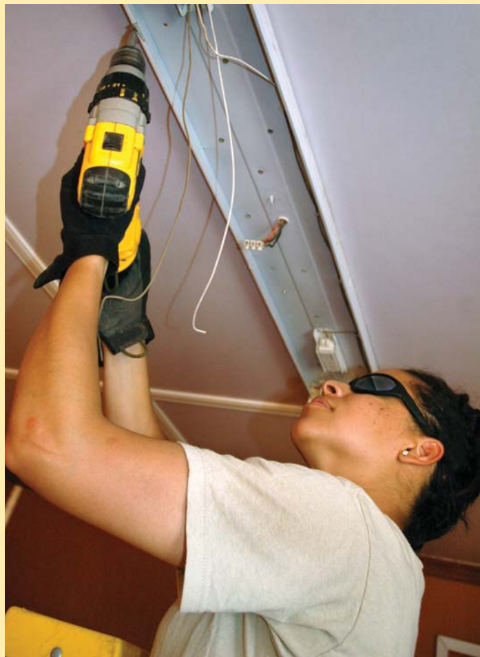
Staff Sgt. Anne McKenzie, Electrician, installs an overhead light fixture in the new Gryphon Air facility.
