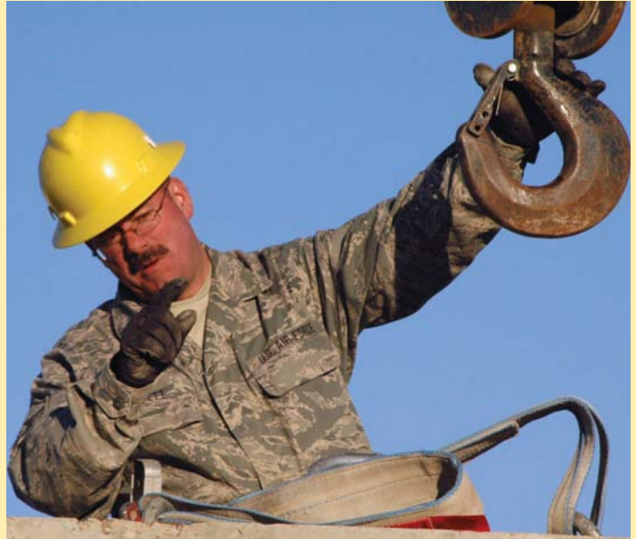
Heavy Equipment Supervisor Master Sgt. Patrick Basnett directs the placement of a "T-wall" barrier in place.
